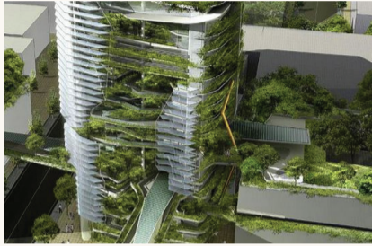
THE GREEN TOWER
